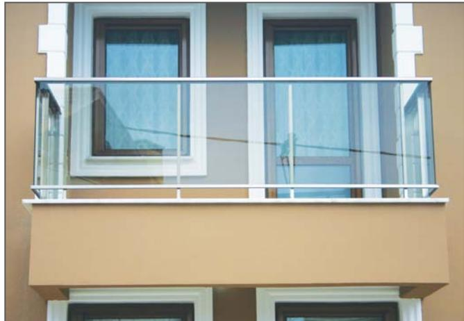
UK **"proton"** is a railing system with rectangular and square profiles which has replaced the traditional systems at balconies, terraces and pools. **"proton"** range of railings will offer you elegance and simplicity at the same time. Most common types of this range have been tested and certified according to 2kN/m horizontal and EN 12600 dynamic (impact) loading.
